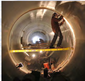
Welding the Lake Hodges Pipeline
