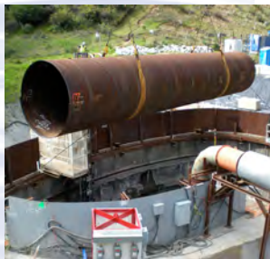
50-foot segment for the San Vicente Pipeline
